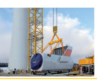
Erection of the hybrid tower of the wind power plant. The crane climbs on its own to a free standing hook height of 93.1 m.
