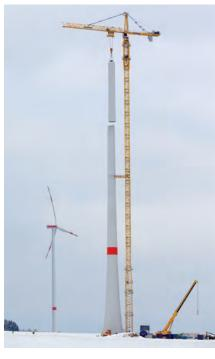
With only one guying arrangement, the tower crane climbs to its final hook height of more than 150 m.
