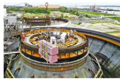
Within four days and three night shifts, the MK 140 lifted a total of 125 tonnes of scaffolding material.
