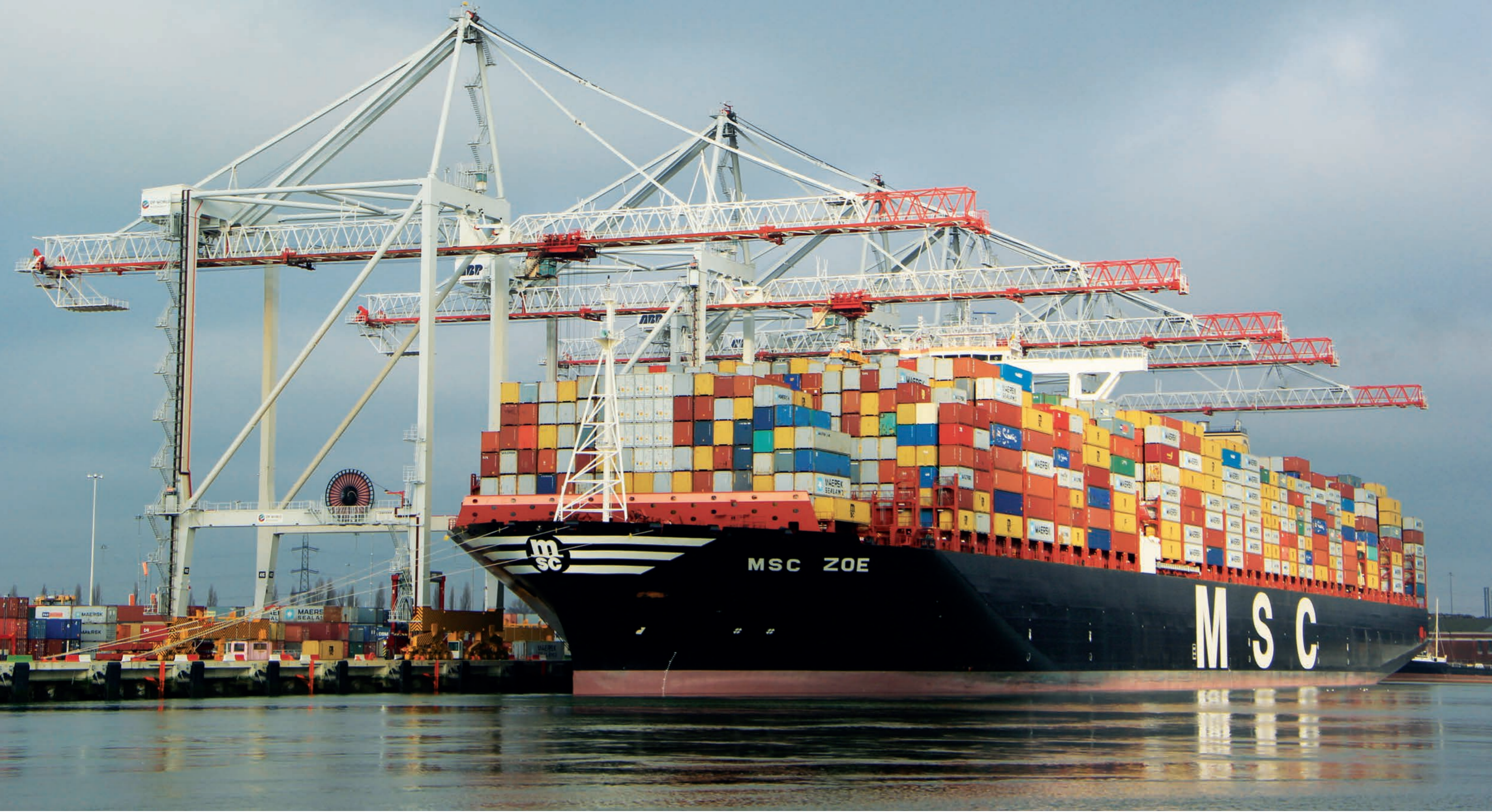
Megamax ship to shore container cranes, Port of Southampton, U.K.
