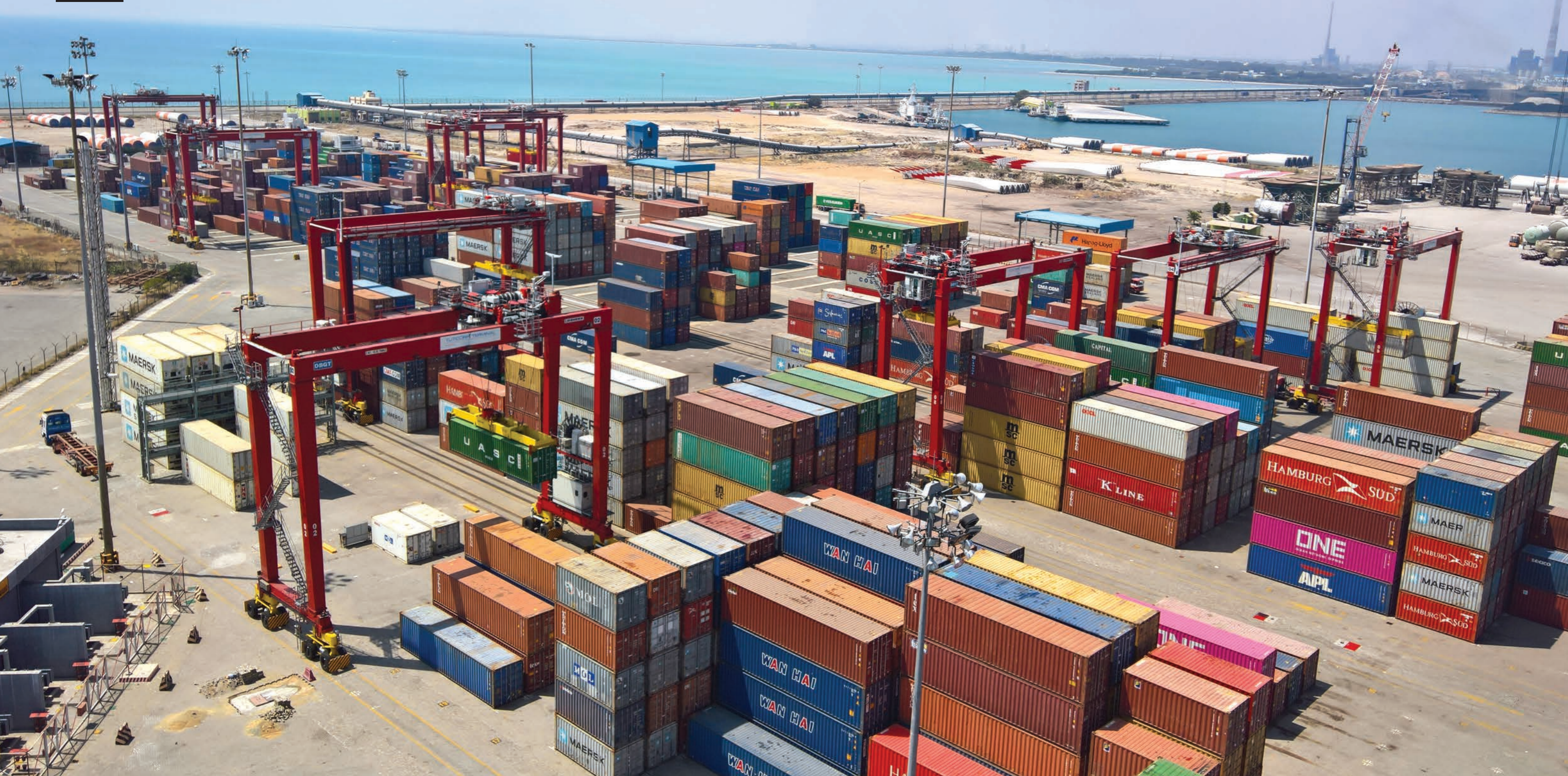
Electric rubber tyre gantry cranes, DBGT, Tuticorin, India.
