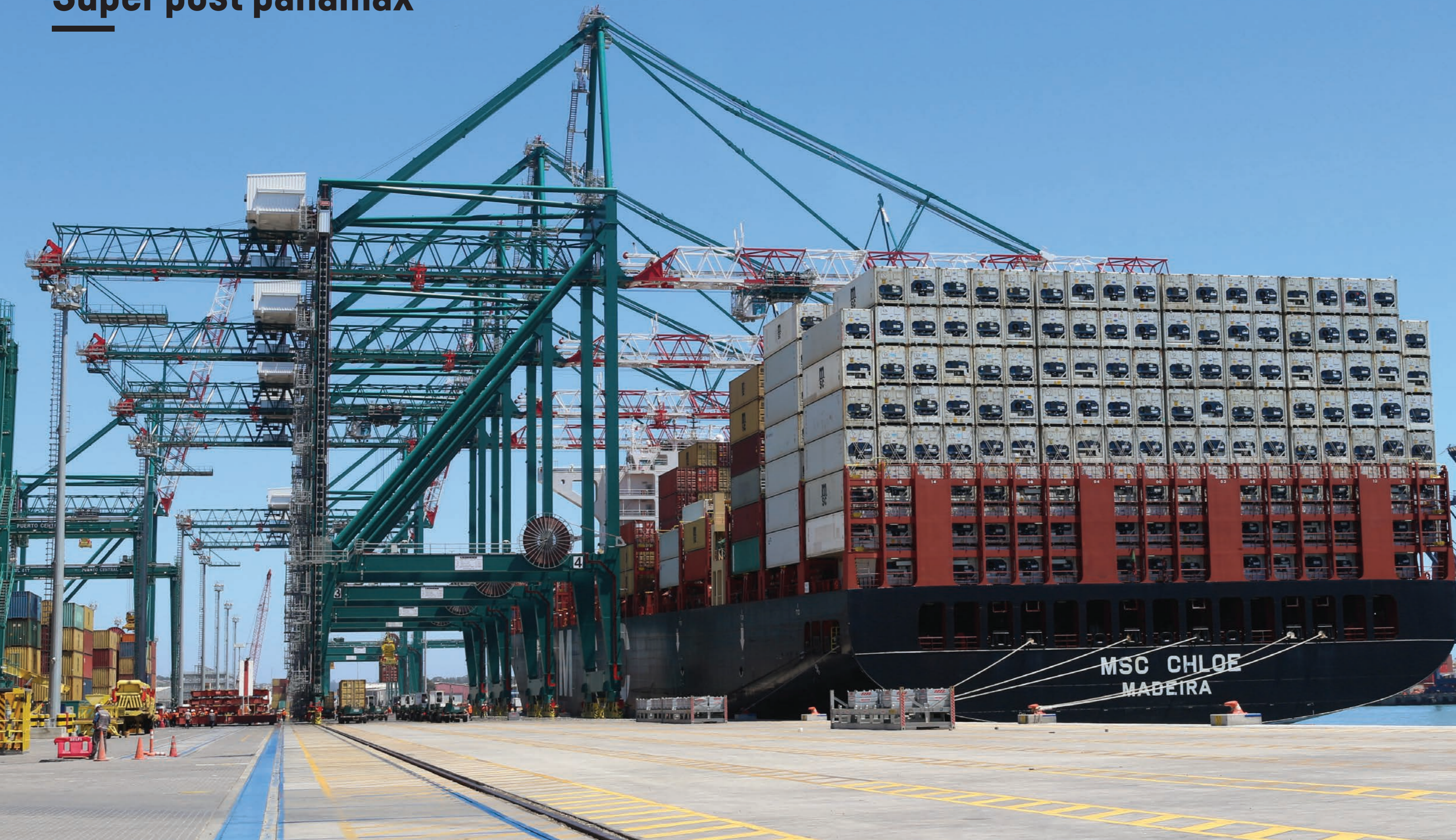
Super post panamax ship to shore container cranes, Puerto Central, San Antonio, Chile
