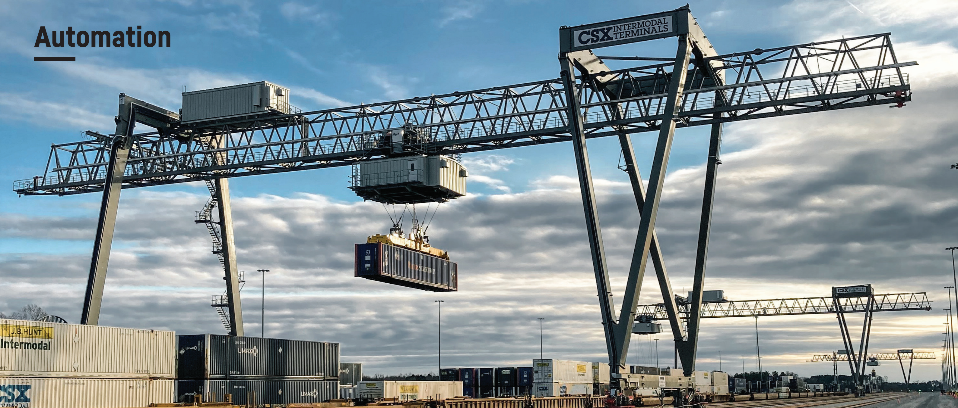
CSX Intermodal Terminals, North Carolina, USA
