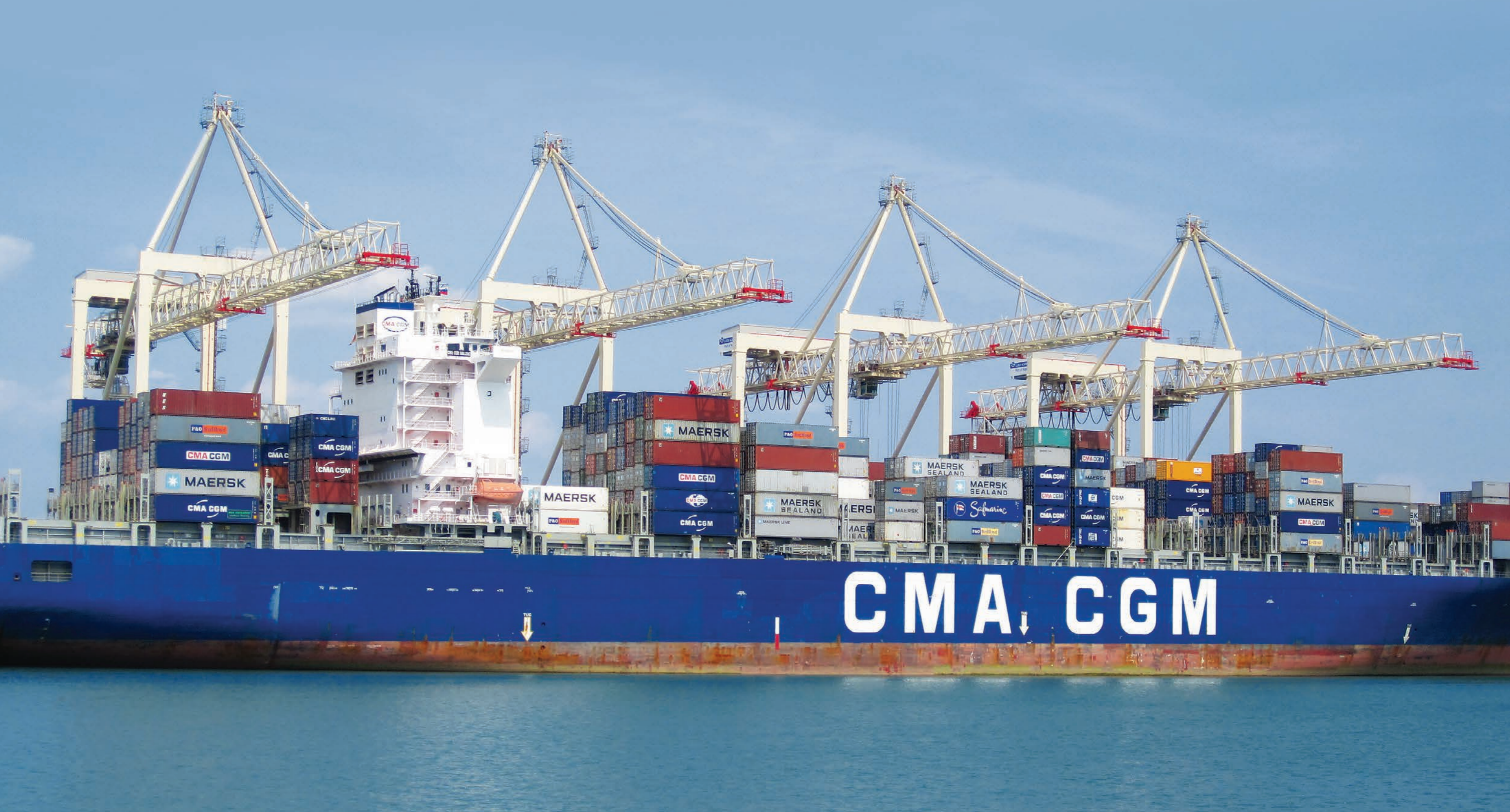
Post panamax ship to shore container cranes, Koper, Slovenia
