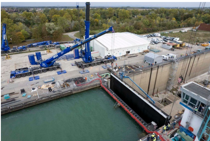
liebherr-ltm-1650-8-1-&-ltm-1450-8-1-msg-06.jpg Precision lifting work right next to the control centre building.
