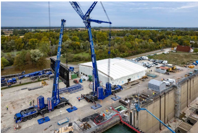
liebherr-ltm-1650-8-1-&-ltm-1450-8-1-msg-02.jpg After being lifted by four mobile cranes, the...
