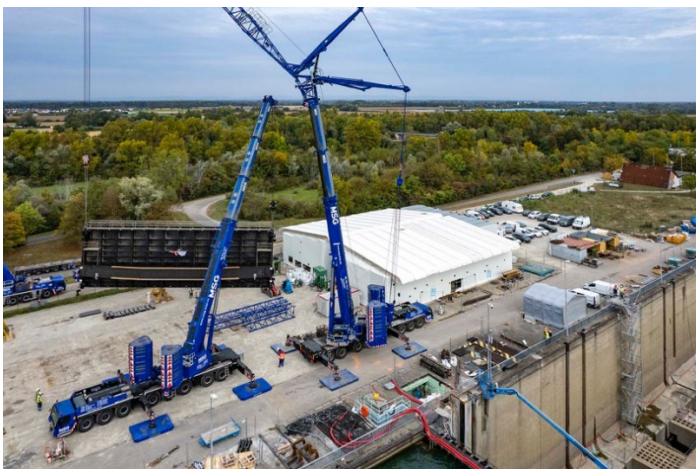
liebherr-ltm-1650-8-1-&-ltm-1450-8-1-msg-03.jpg ... barrier gate is first turned by the Liebherr cranes...
