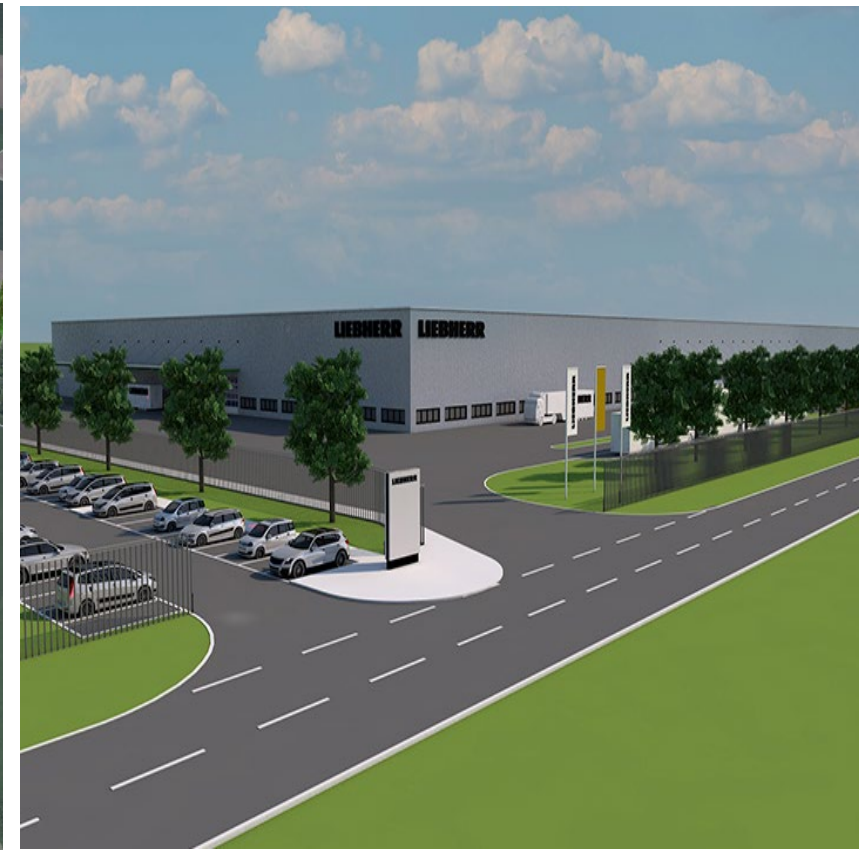
Namsheim, France: new manufacturing site for welded components, (pre)-assembly work for cabs
