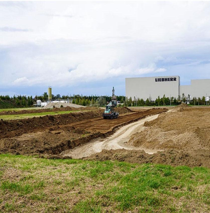
Oberopfingen, Germany: expansion of the hydraulic cylinder plant and central logistics
