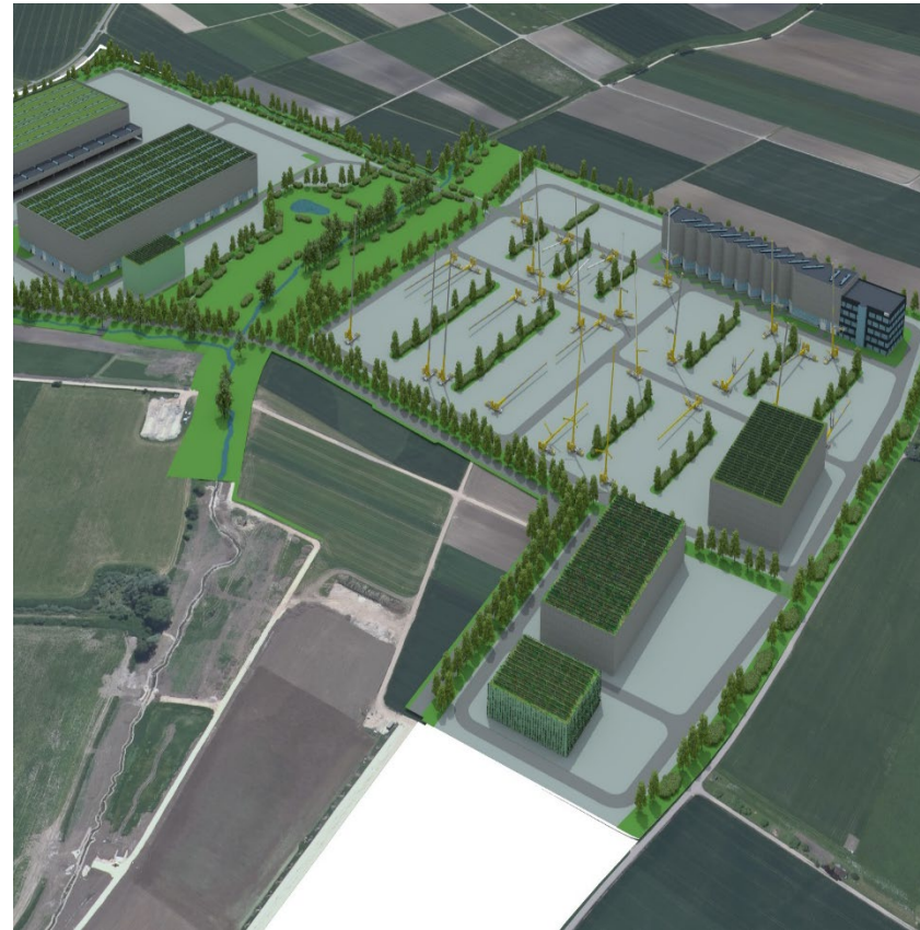
Echingen, Germany: Plant expansion for mobile and crawler cranes
