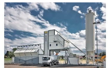
New concrete mixing plants
