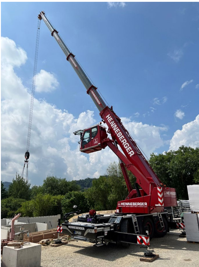
liebherr-ltc1050-3-1-henneberger-ilmenau.jpg The LTC 1050-3.1 assembles wall elements in Ilmenau.
