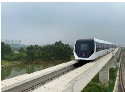
chengdu-xinzhru-road-and-bridge-machinery-maglev-train.jpg Maglev train project by Chengdu Xinzhru Road & Bridge Machinery Co., Ltd.- © Max Boegl
