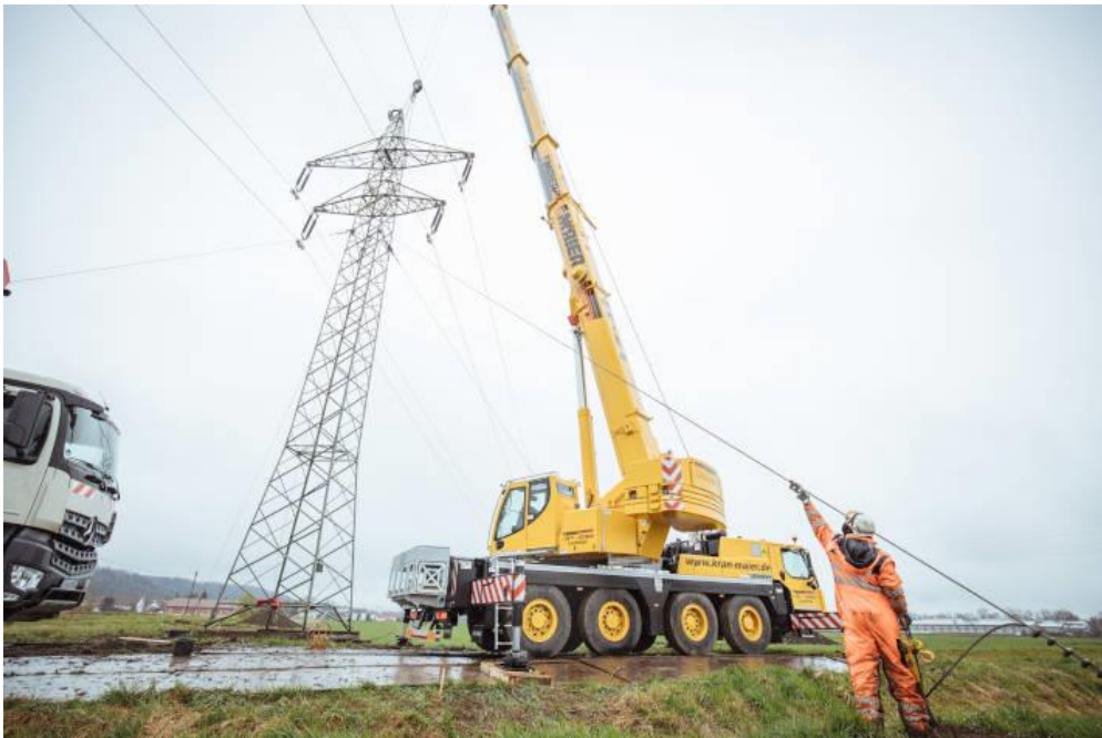
liebherr-ltm1070-4-2-maier-motive02.jpg The new poles are built on the existing foundations.
