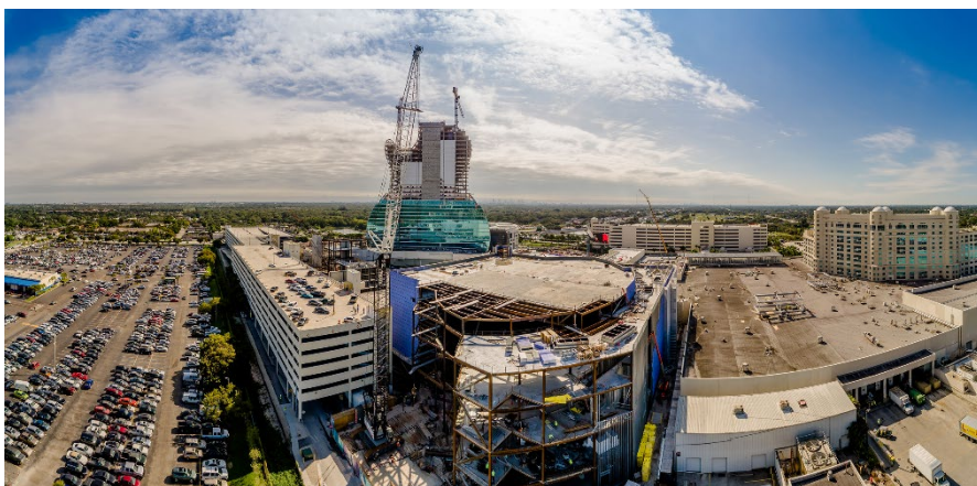
liebherr-lr1300.jpg Liebherr crawler crane LR 1300 operating in Florida, United States.
