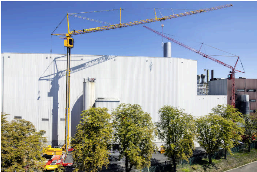
liebherr-mk88-mk140.jpg MK88 and MK 140 on an industrial installation job.
