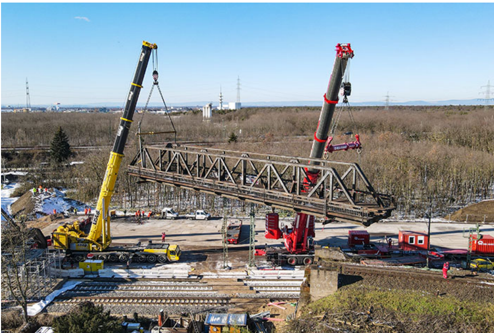
liebherr-riga-ltm1650-8.1-eisele-ltm-1500-8.1-motive02.jpg Sensitive – the massive load is slewed carefully between the two cranes so it can be placed on SPMTs.
