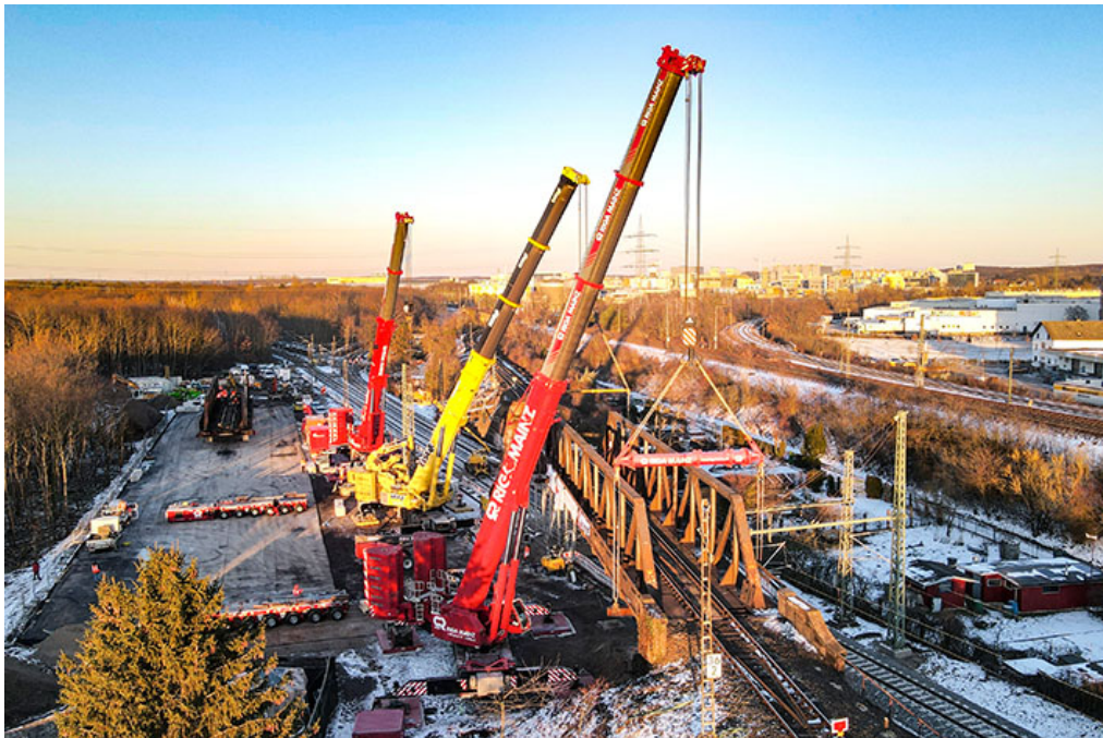
liebherr-riga-ltm1450-8.1-eisele-ltm-1500-8.1.jpg Bridge number 2 – Riga's LTM 1450-8.1 in tandem with Eisele's LTM 1500.8.1 remove the same weight at a slightly lower radius.
