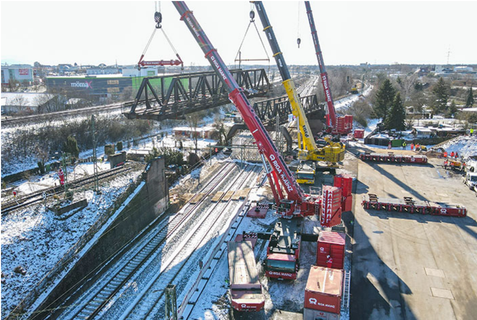
liebherr-riga-ltm1650-8.1-eisele-ltm-1500-8.1-motive01.jpg 160 tonnes on the hook – bridge number 1 is suspended on the hooks of Riga Mainz's LTM 1650-8.1 and Eisele's LTM 1500-8.1.
