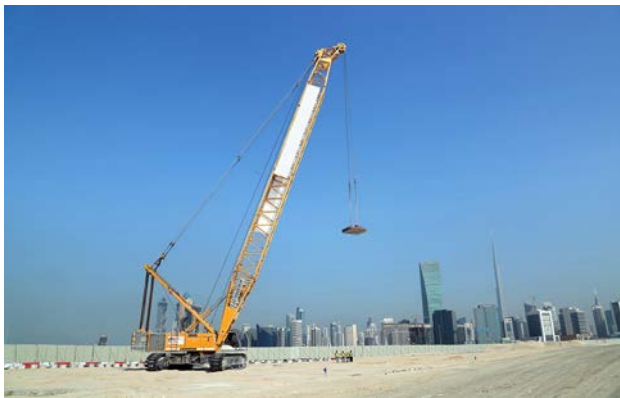
liebherr-o.rentals-dubai.jpg Deep soil compaction in Dubai.
