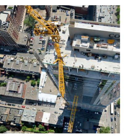
The derrick crane was ideal for the very restricted space available on the roof of the hotel: reliable and safe dismantling of the Liebherr 355 HC-L 12/24 Litronic luffing jib crane.
