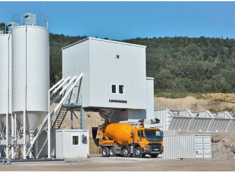
The horizontal concrete mixing plants in the Betomix series are of modular design. With outputs as high as 210 m<sup>3</sup> set volume of concrete per hour, the Betomix has the performance to satisfy every need.
