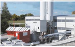
Compactmix 1.0 with cladding, affiliated to a prefabricated plant
