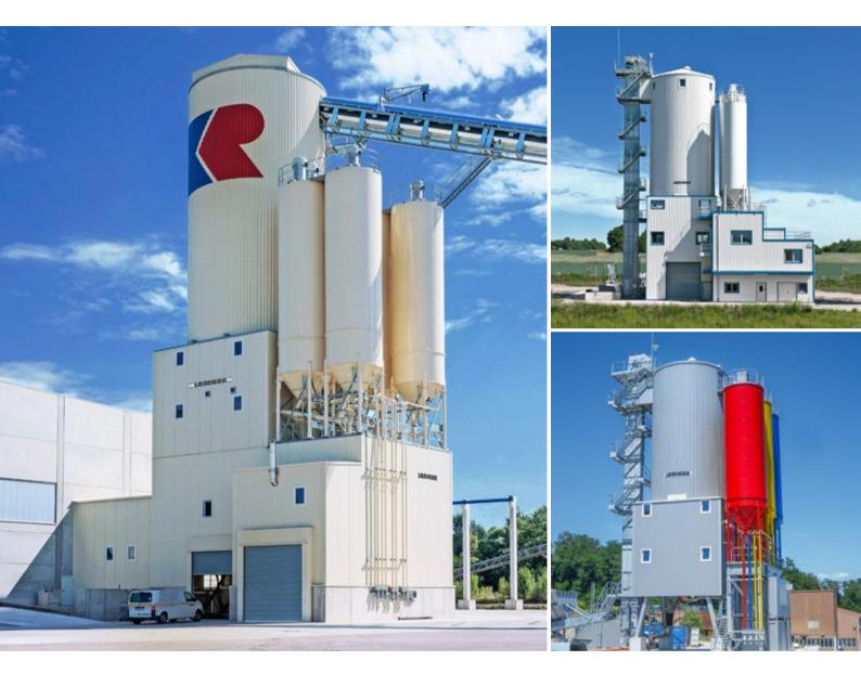
For many years Betomat-type tower plants have been used successfully all over the world for pre-mixed concrete as well as in the prefabricated and pre-cast element production industries.
