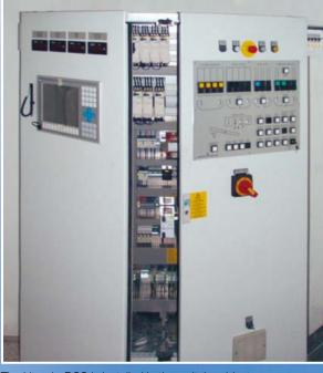
The Litronic-BCS is installed in the switch cabinet to save space.
