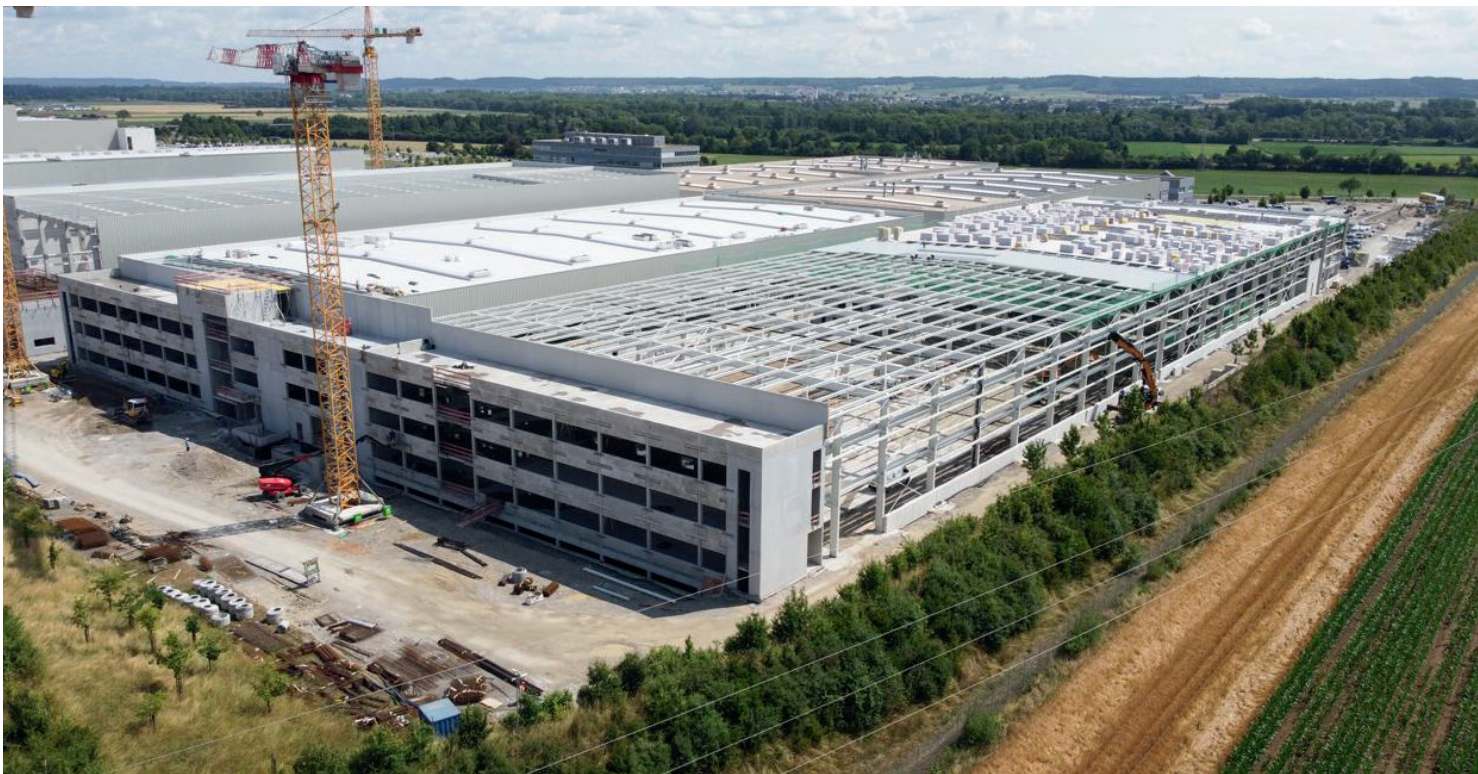
Figure 9: Implementation status of the new building in summer 2023: Three new halls for mechanical production, logistics and other areas as well as an additional administration building are being built on 46,000 square metres. In the background are the buildings that have been in use since 2017 for assembly, paintwork and administration.
