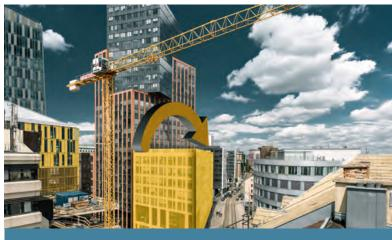
3D ABB: By factoring in the lowering depth, the working range limiting system becomes three-dimensional. This makes it possible to negotiate low protected buildings and to reach working areas under protected structures.
