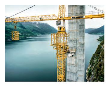
Activating climbing mode automatically limits crane operation, converting it to a special climbing load curve. This enables the climbing to be carried out safely, while reducing hazards due to improper actions.
