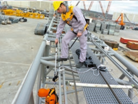
Positioning the karabiner with the aid of a telescopic rod
