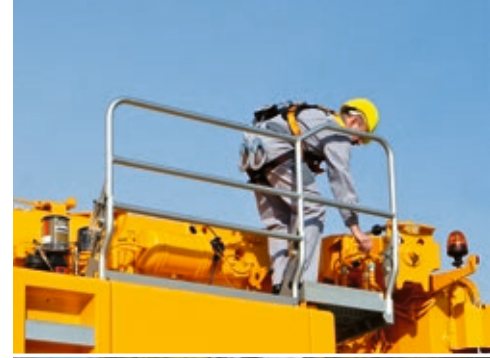
Securing by railings
