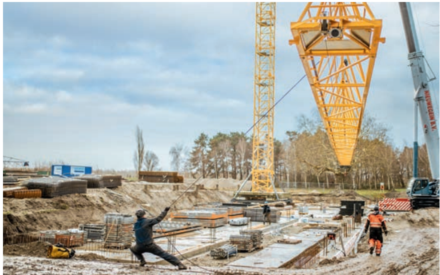
The wind is a force to be reckoned with while assembling the jibs
