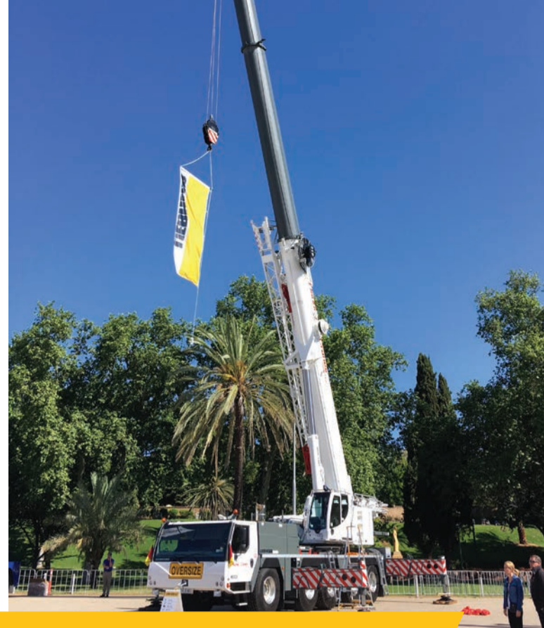
» Fleurieu Cranes' Liebherr LTM 1130-5.1 on display at CICA.
