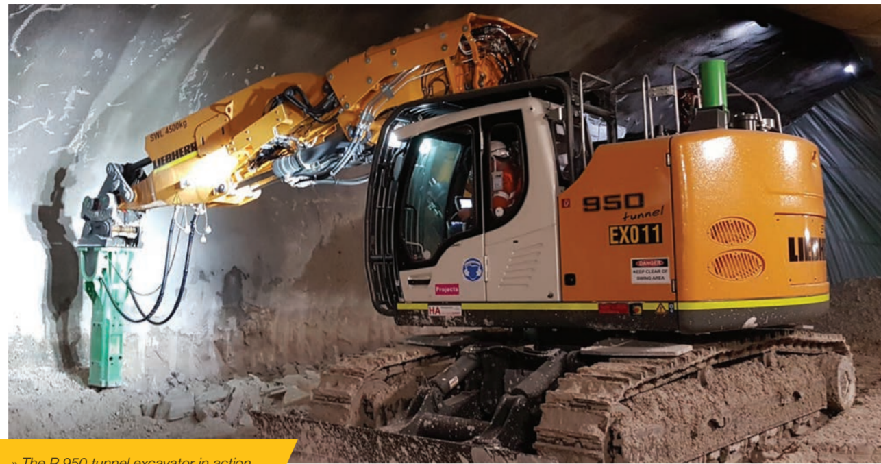
= The R 950 tunnel excavator in action.
