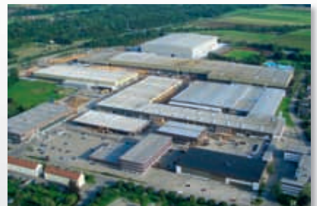
Kirchdorf: hydraulic cylinders
