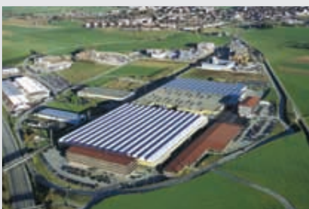
Bulle: diesel engines, splitter boxes, hydraulics
