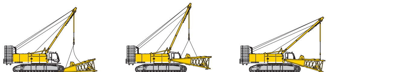
Unloading and assembly of boom foot
