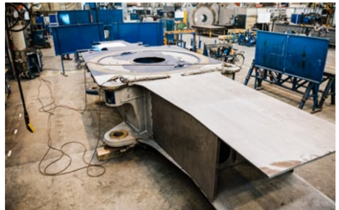
Preparation of a frame section for repairs after an accident
