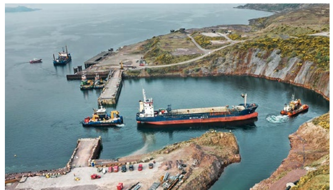
With an area measuring 160 by 160 metres, the dry dock has plenty of space for large freighters like the MV Kaami.
