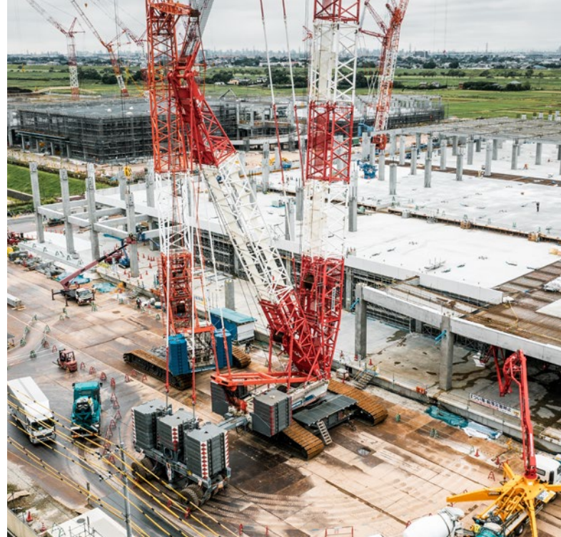
Fast relocation of the cranes on site using the ballast wagon
