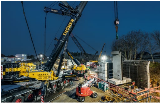
All done The reinforced steel elements used to assemble the modular abutments weighed up to 92 tonnes. They are shown here on the hook of the LTM 1750-9.1.
