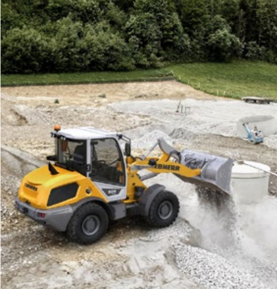
The L 506 in site work
