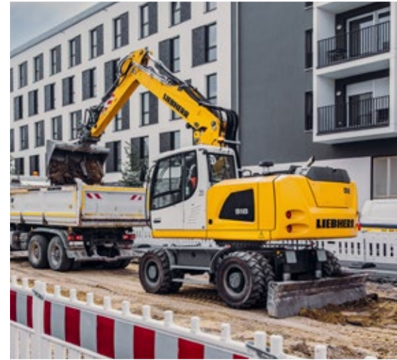
The A 918 Litronic for earthmoving work in Regensburg (Germany)
