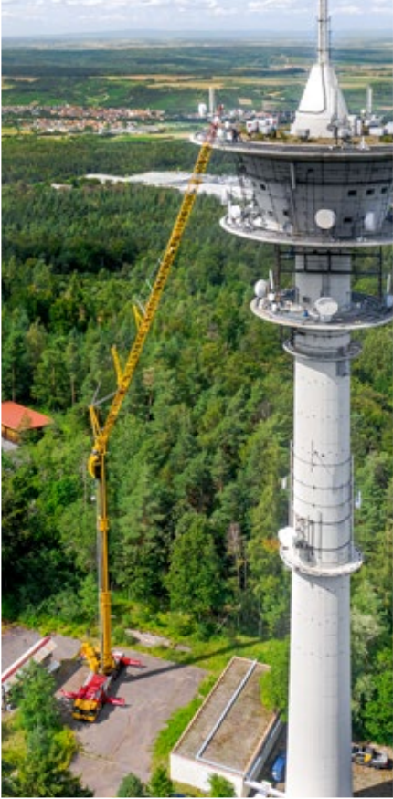
The MK 140 in luffing mode during the exchange of antenna technology of a telecommunications tower
