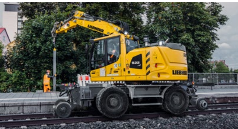
The A 922 Rail Litronic used for installing a noise barrier
