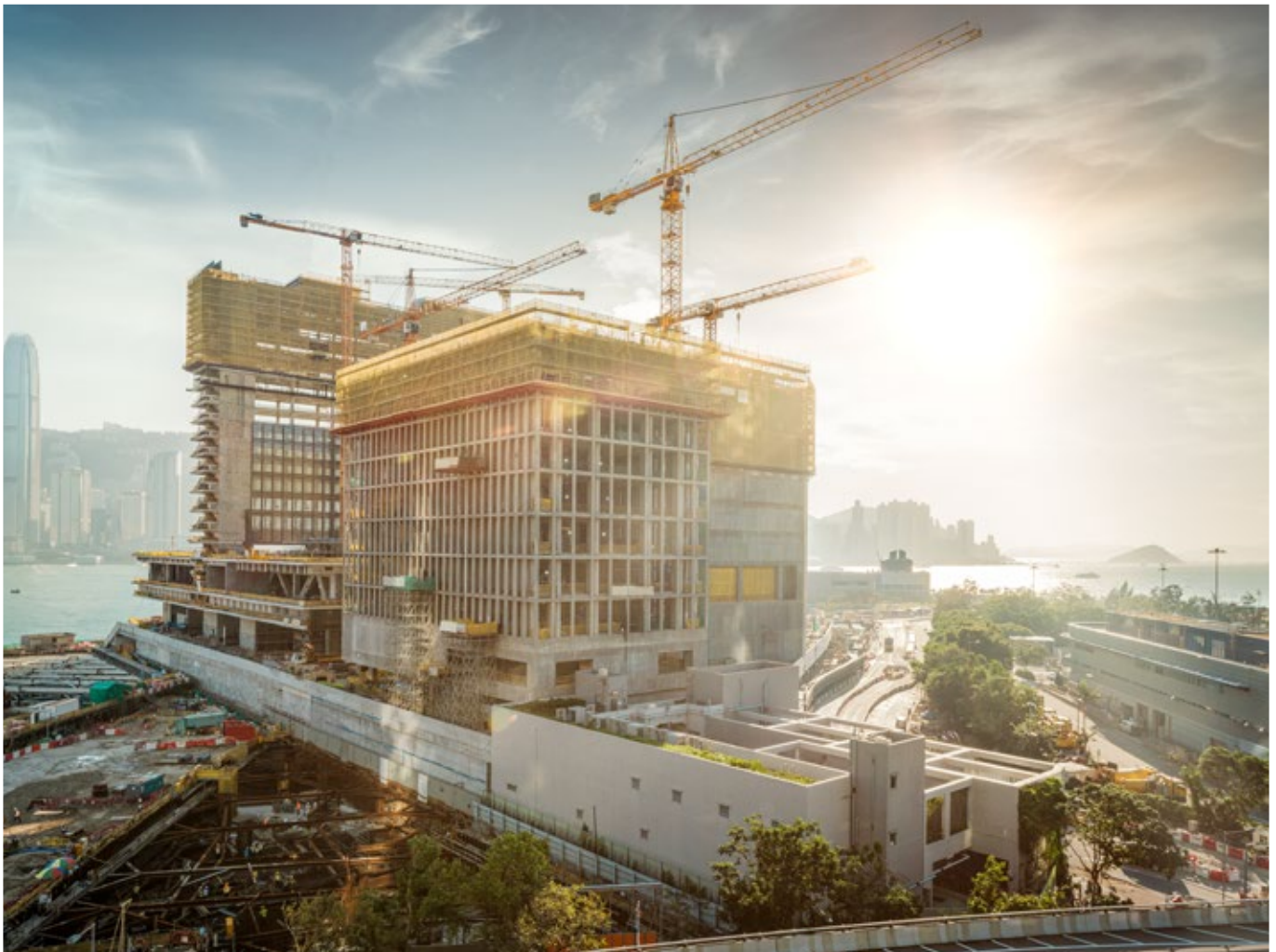
Serving culture and education: Top-slewing cranes used in the construction of the M+ museum in Hong Kong (China)
