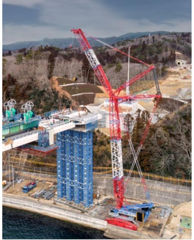
A LR 1750/2 used for a bridge construction in Japan
