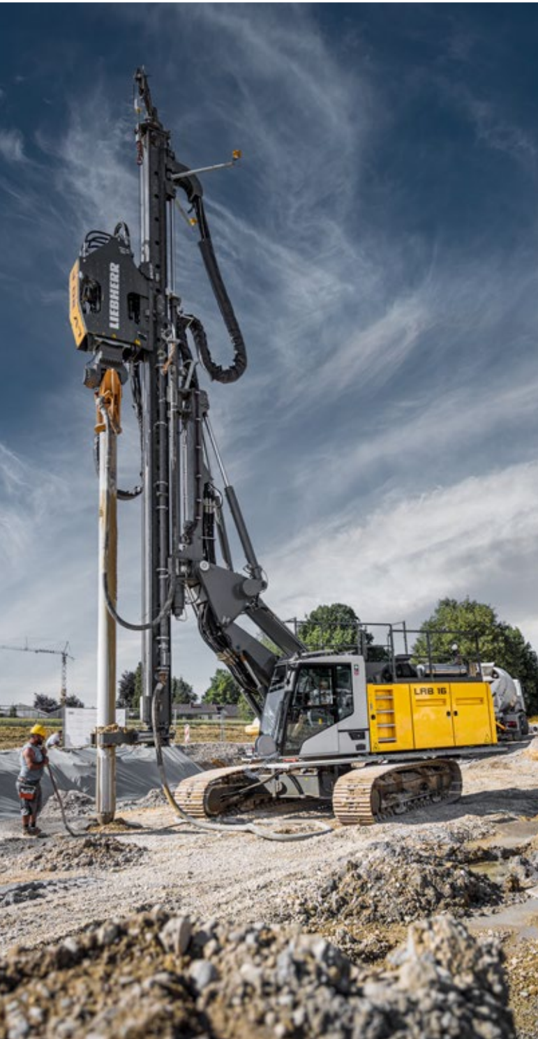
The piling and drilling rig LRB 16 installing cast-in-place vibration piles
