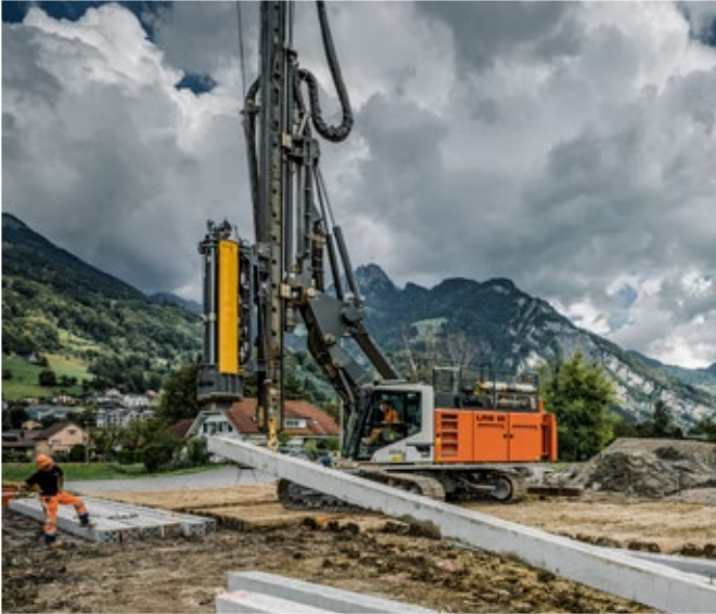
The LRB 18 driving precast concrete piles at Lake Walen (Switzerland)
