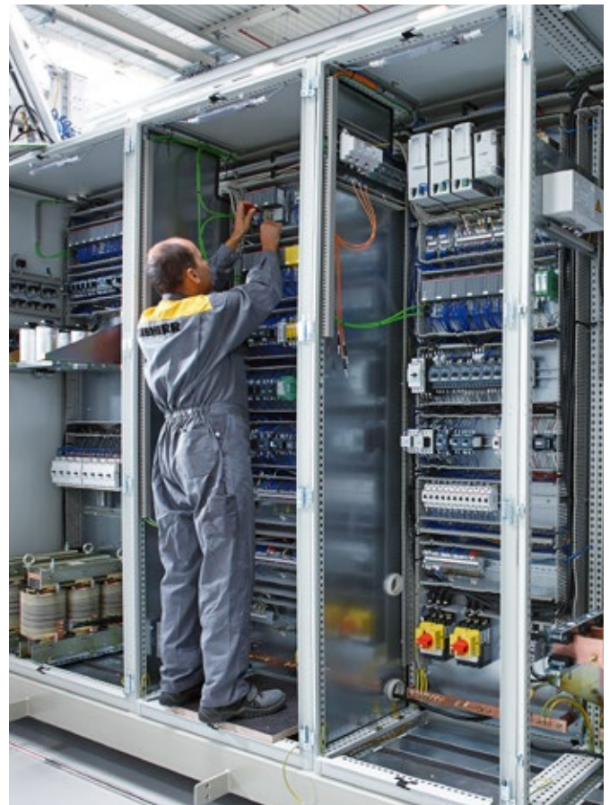
Installation of control cabinets for container cranes
