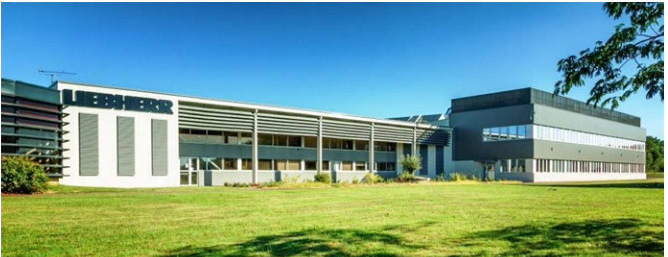
The expansion of the Campsas site will help to increase production capacities by up to 30 percent in the years to come.
