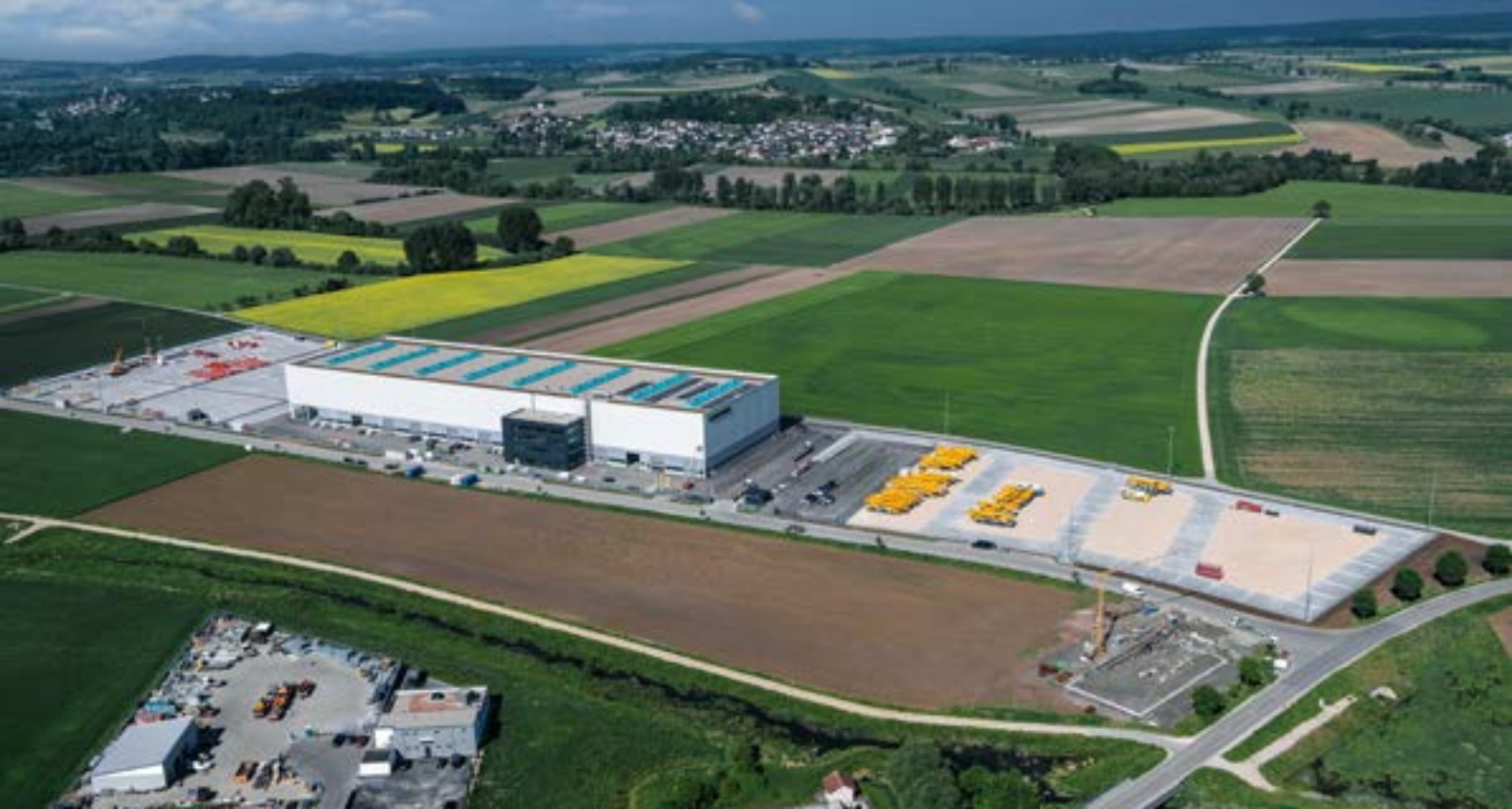
The repair centre at the Ehingen-Berg site.
