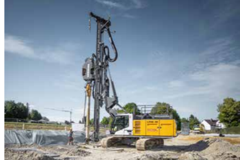
Deep foundation machines
