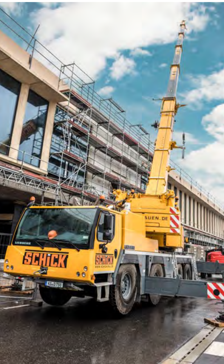
An LTM 1090-4.2 installs coloured concrete façade elements on Pier H.
