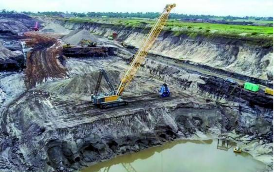
The HS 985 HD in a sand quarry in Lang Lang, Victoria. ▶
