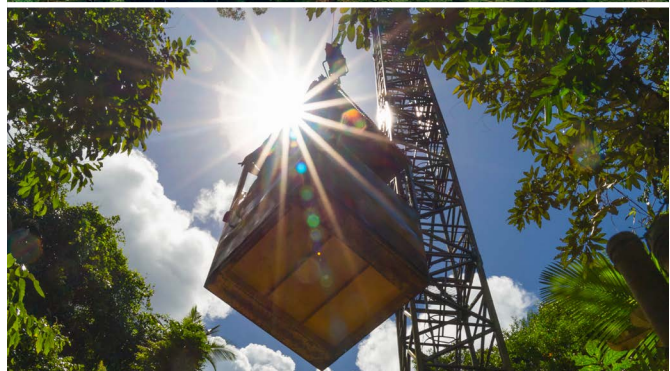
The longest standing crane in Australia, a Liebherr 91EC.
