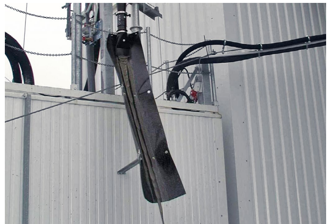
Hydro-cyclone The hydro-cyclone reduces the amount of solids in the residual water.
