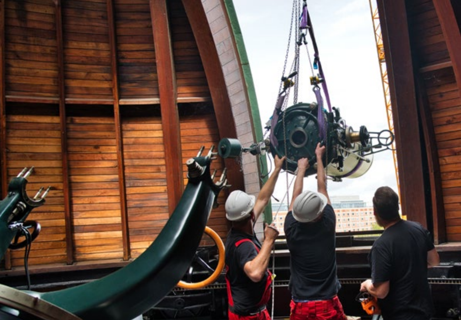
Made to measure – Museum staff align the telescope with centimetre precision so that it can be lifted out through the slit gate of the East Observatory.
