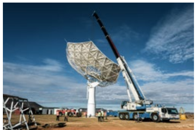
The LTM 1220-5.2 assembling the SKA MPG prototype antenna in the Karoo, South Africa. Image: Nasief Manie/SARAO
