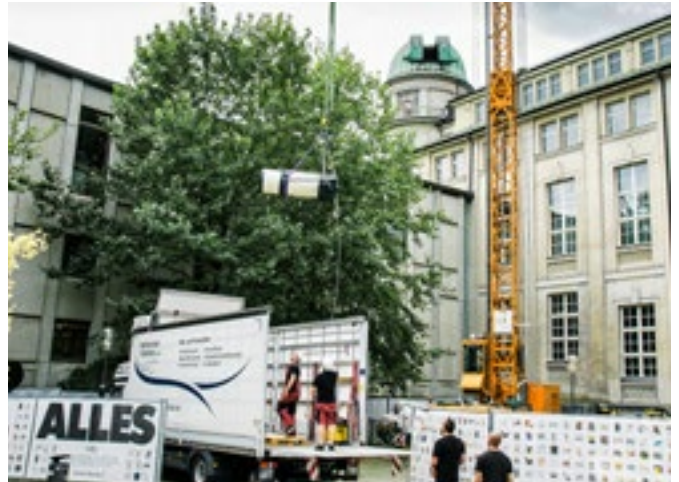
The Treffler MK 88 carefully lifts the Goerz telescope from the observatory of the Deutsches Museum into the transport vehicle. Image: Bernhard Thaler
