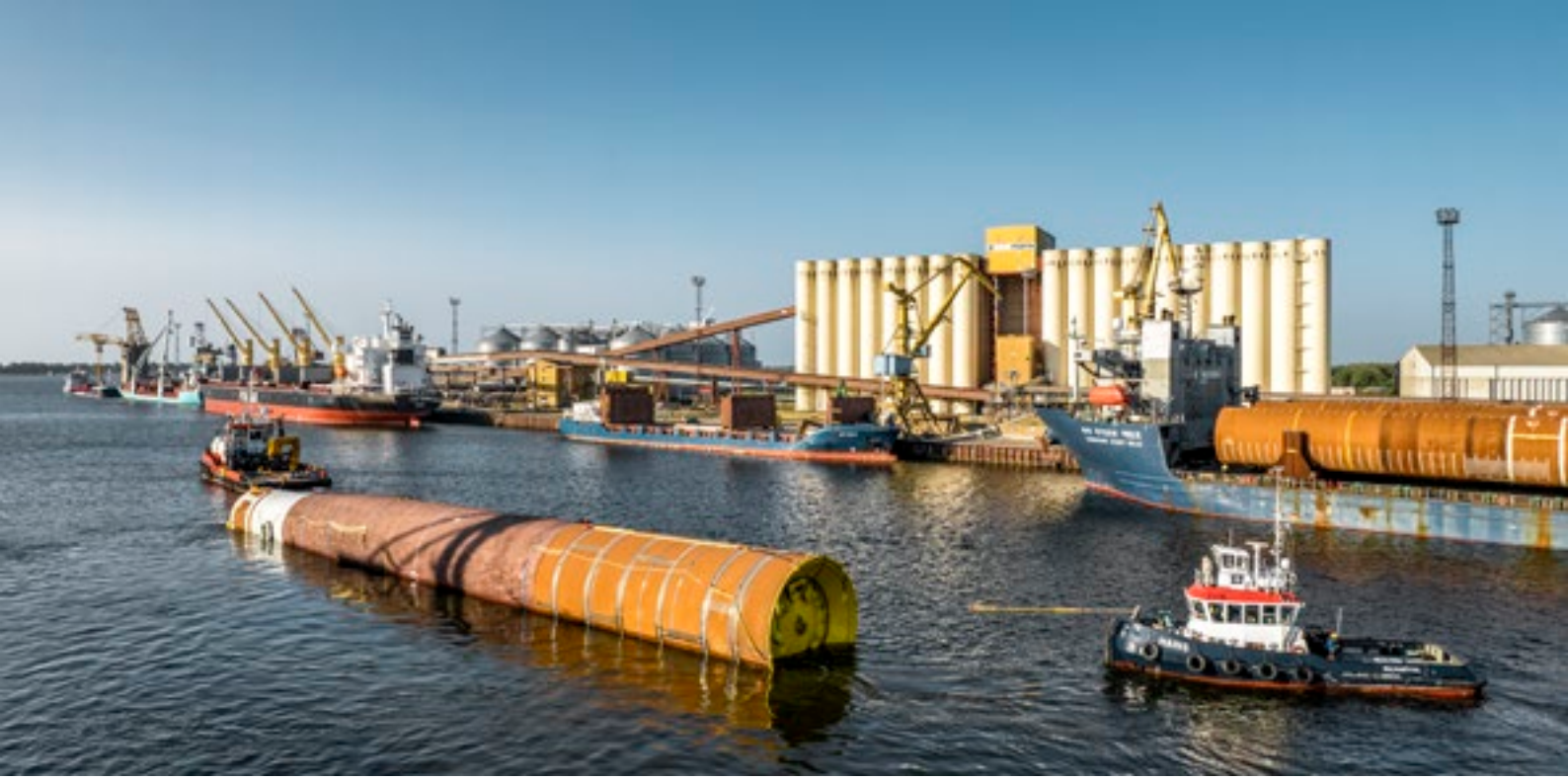
So here we go. A tug tows the floating monopile into the Baltic Sea. The 85 nautical mile journey to the offshore construction site takes 15 hours.
