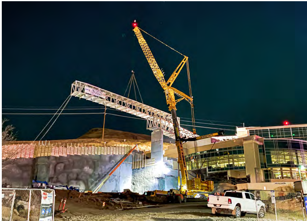
The upgraded LTM 1750-9.1 delivers sufficient power in reserve for the job in Utah.
