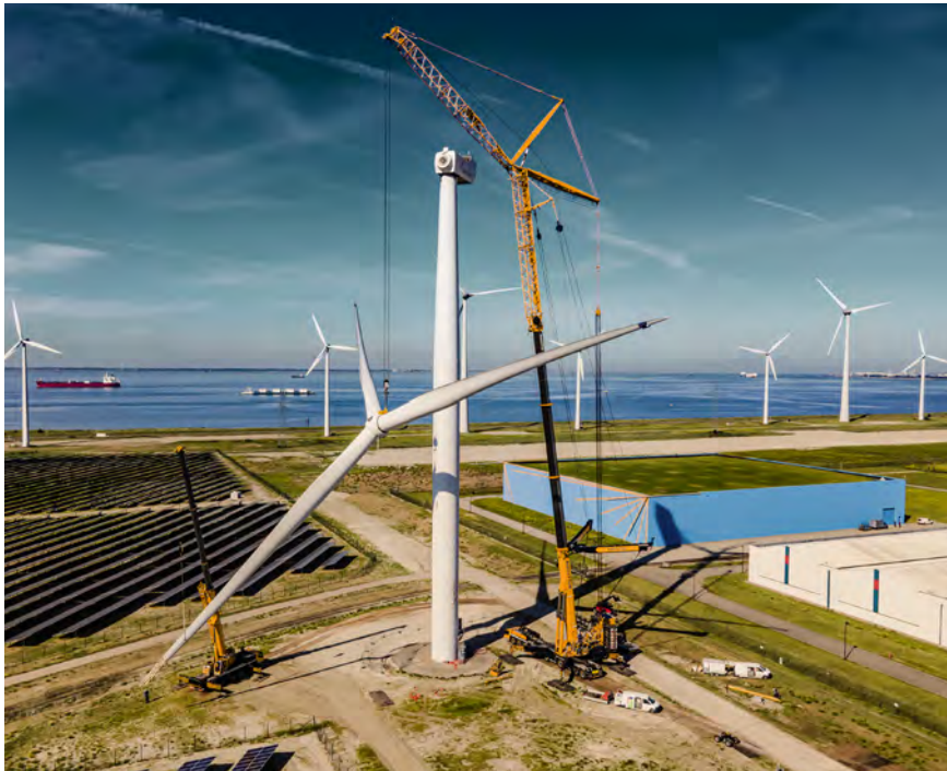
Dismantling a wind turbine in the Netherlands.
