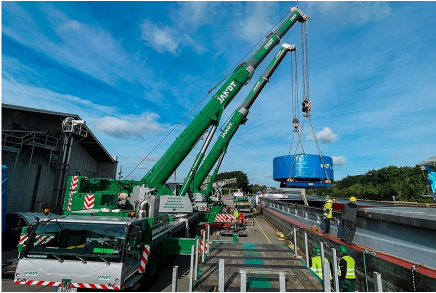
liebherr-ltm1250-5.1-jandt-03.jpg At 98 tonnes, the generator was the heaviest component.
