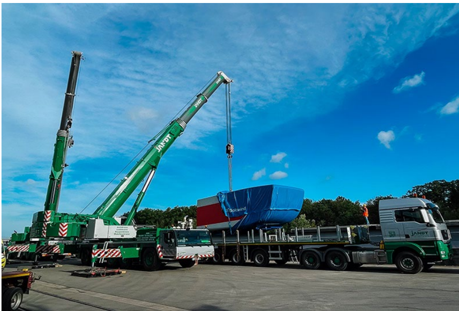
liebherr-ltm1250-5.1-jandt-04.jpg An LTM 1250-5.1 is sufficient for loading the lighter nacelle.
