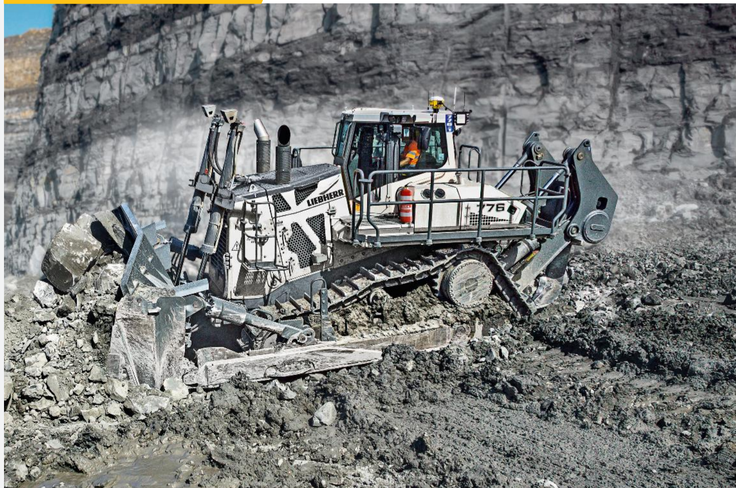
» The PR 776 working with the R 9800 excavator.
